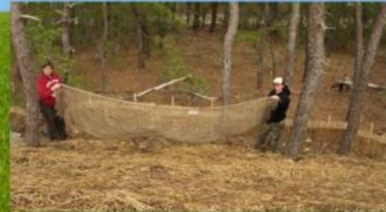
Jute netting and ground staples will help secure slope materials.
