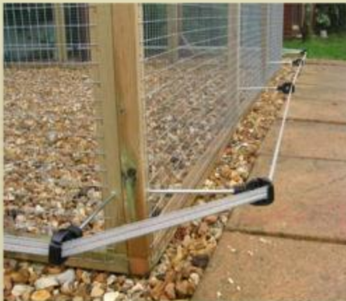
Single line electric fence around the exterior wall
