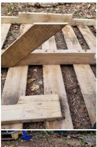
8. Align the end of the support beam to the edge of the first reinforcement plank
