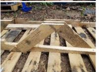
9. Repeat on the opposite side to form a triangle with a second connecting plank
