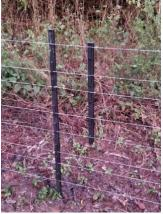
4. If the string is touching metal, is in close proximity to a tree, or is touching another grounding source, move the wire or wrap in electrical tape to prevent electricity drain
